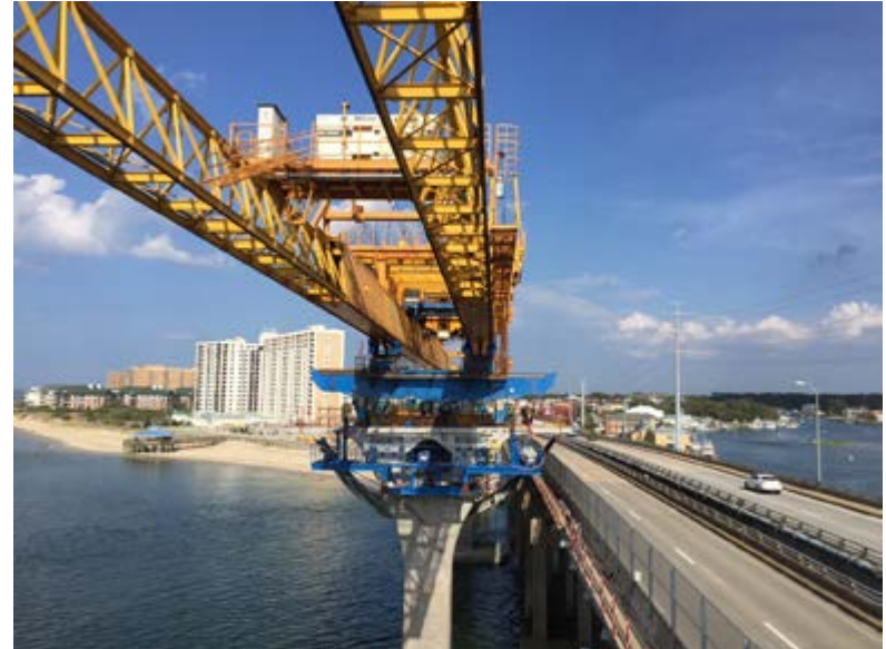
Lesner Bridge under construction (above) and finished (left).
