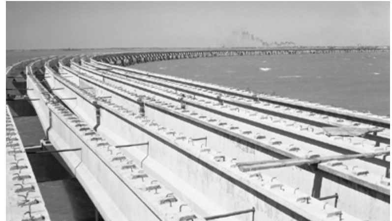
Hampton Roads Bridge Tunnel under construction (above) and finished (left).
