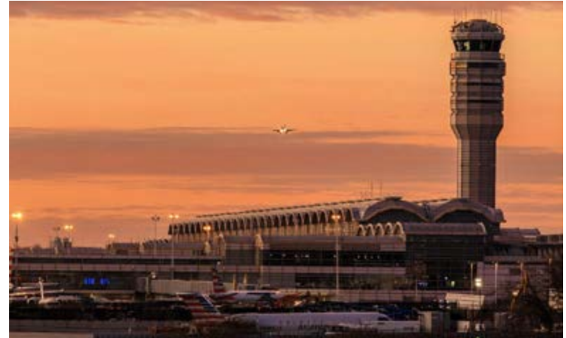
Airport interior (left) and expansion (above).
