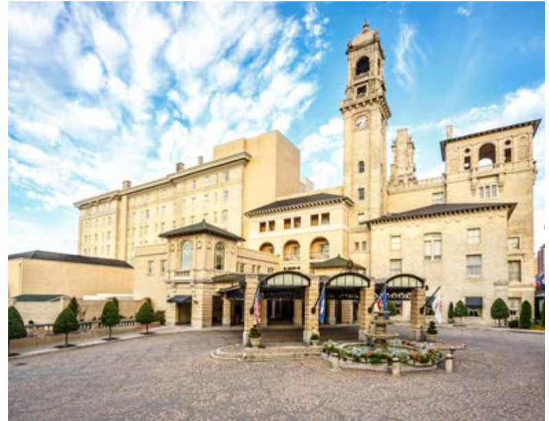
The hotel's Franklin Street entrance (above) and interior restoration (right).
